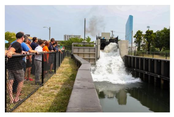
Image: Underground flood control infrastructure (Baltic Avenue Canal) at Fisherman's Park in Atlantic City. Water drains from 775 acre of Streets into the canal to alleviate flooding. Photo Courtesy: Kristian Gonyea/The Press of Atlantic City
